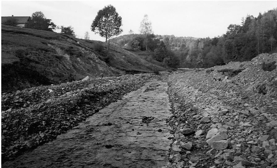
Fig. 6. The Kamionka stream channel after the 1997 flood
